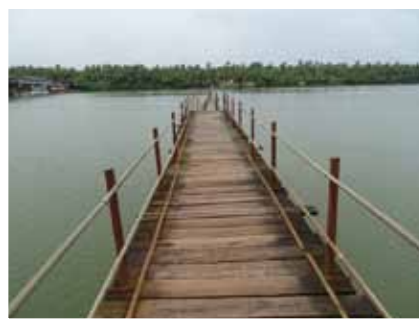
Kottapuram - Achamthuruthi Foot Bridge
