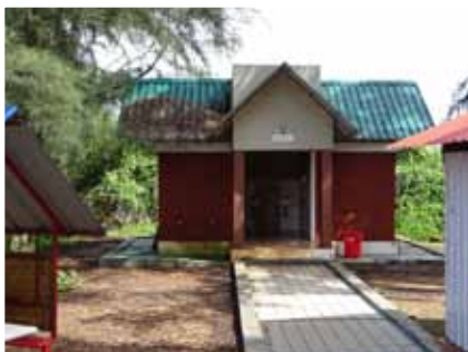
Toilet block, Chootad beach park
