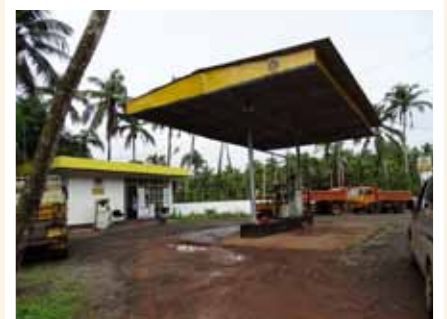
Fuel Station at Thuruthi
