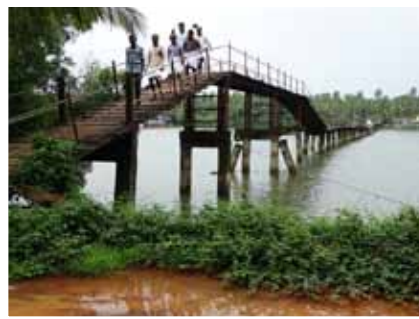
Walking Bridge over Kottapuram
