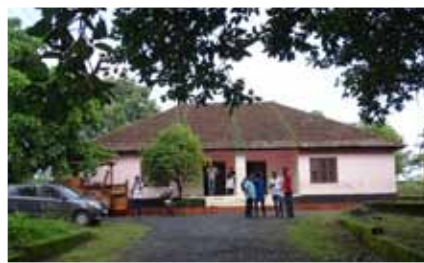
Water Authority guest house, Madayi
