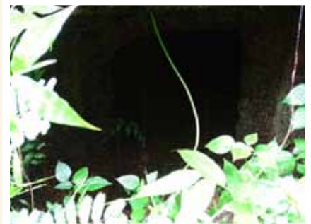
An underground tunnel
