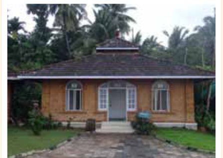
Toilet block at Sargaalaya
