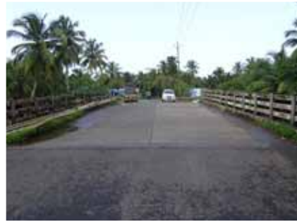
Sultan Canal Bridge
