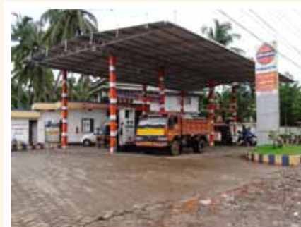
Fuel Station, Padanna
