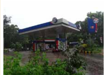
Fuel Station, Edayar
